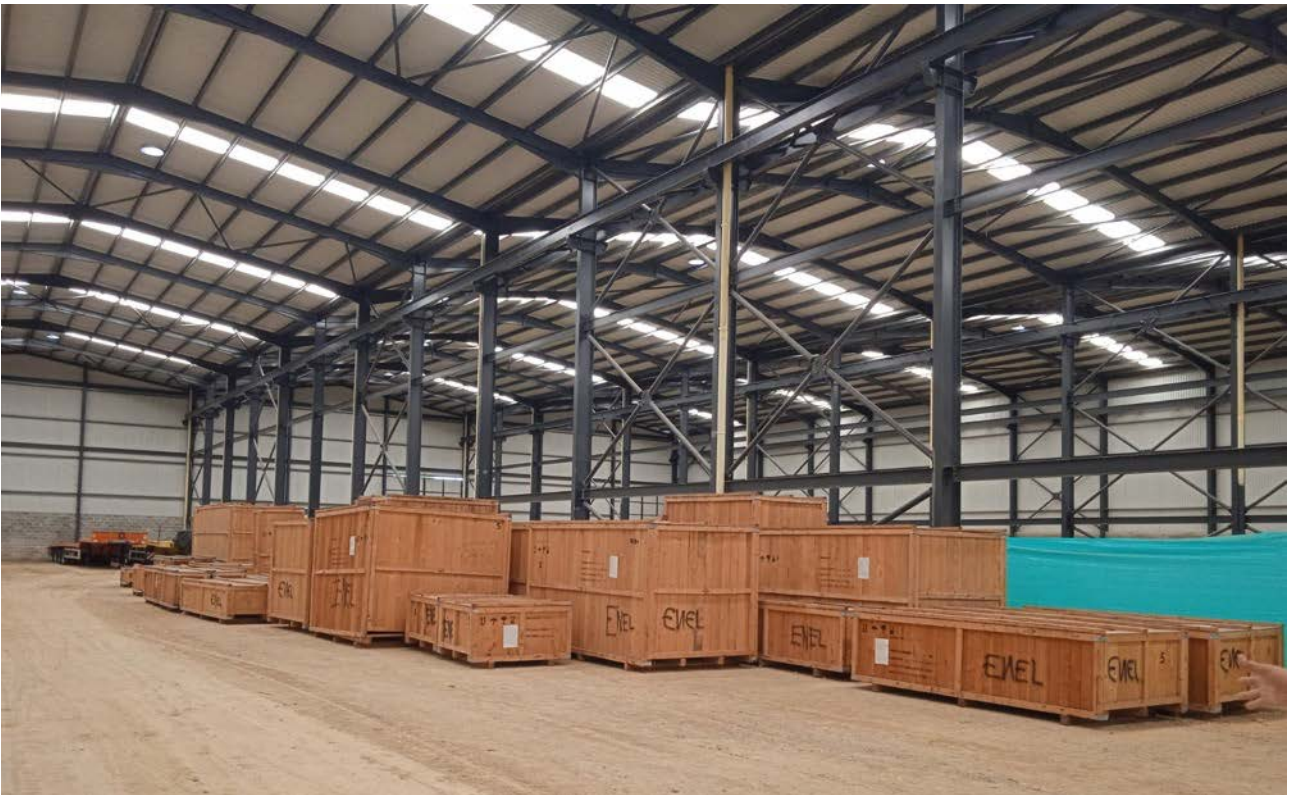
Figure 15: Substation parts storage status 4
