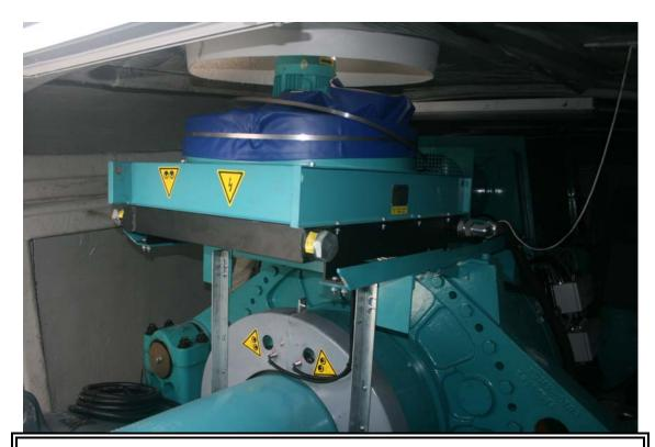
Figure 17 Oil cooler forward of gearbox with blue flex duct separated from nacelle.
