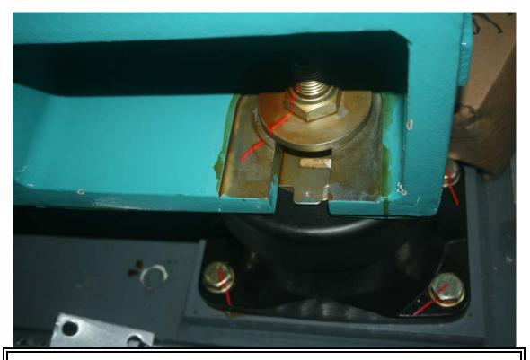
Figure 45 Right front generator mount. Generator frame attachment bolting not moved. Elastomeric insert bolting moved.
