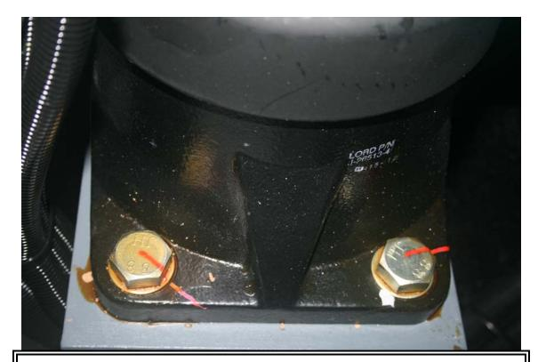
Figure 39 Left rear generator mount. Generator frame attachment bolting not moved.
