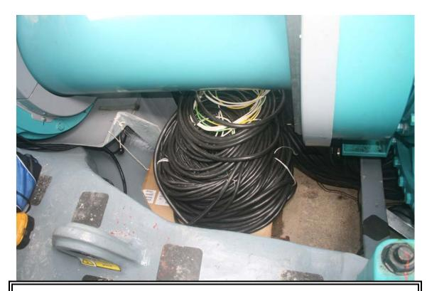
Figure 21 Tower cables coiled below main shaft viewed from the left side.
