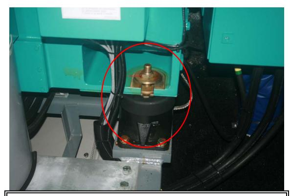
Figure 38 Left rear generator mount.
