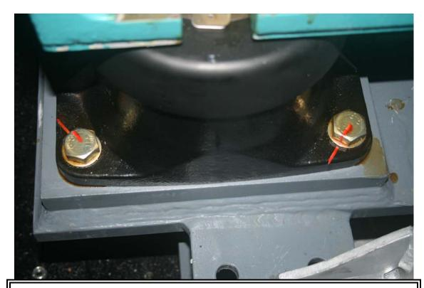
Figure 43 Right rear generator mount. Generator frame attachment bolting not moved.
