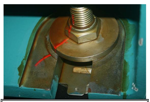
Figure 46 Right front generator mount. Elastomeric insert bolting moved.
